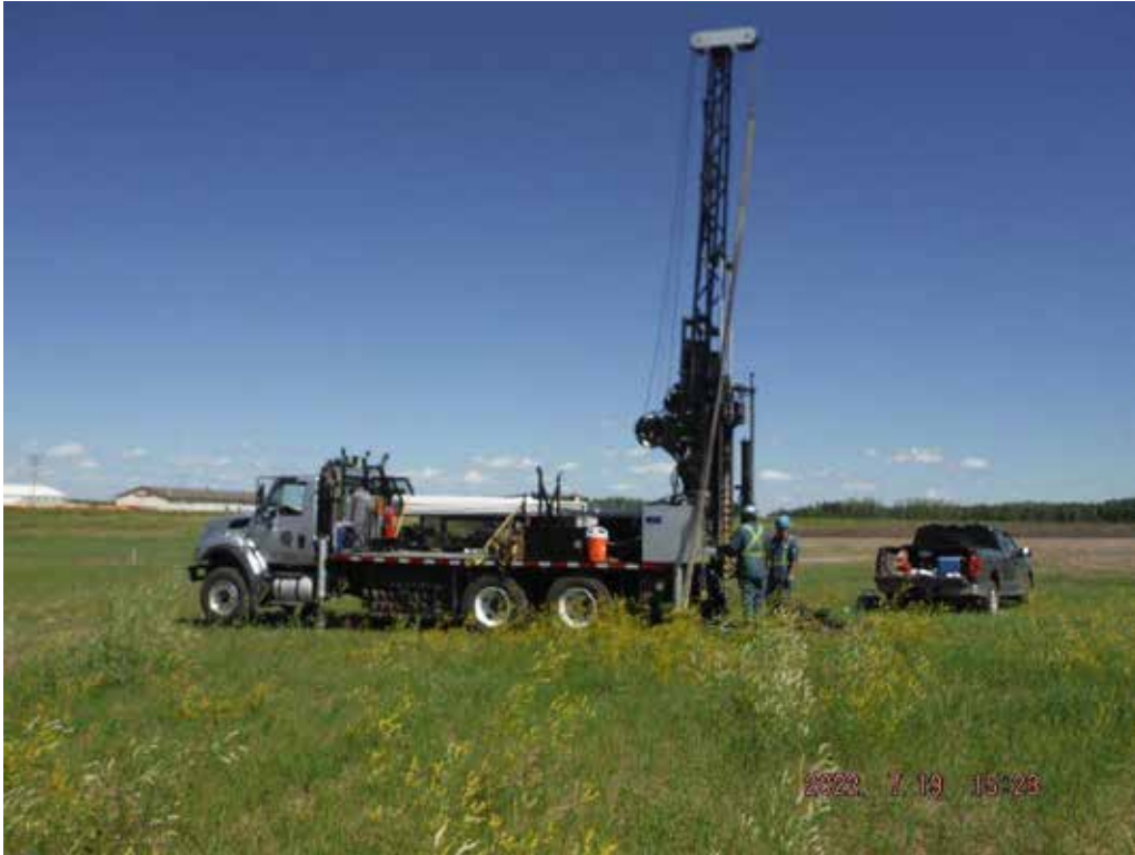
Photograph 1: Looking east during the drilling of BH22-02
