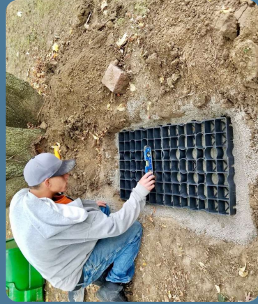
Figure 37: Grade Beam Alternative, Source: MonuGrid Concrete ReplACEMENT
