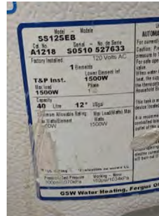
Figure 4-9 Electric Water Heater Nameplate Data
