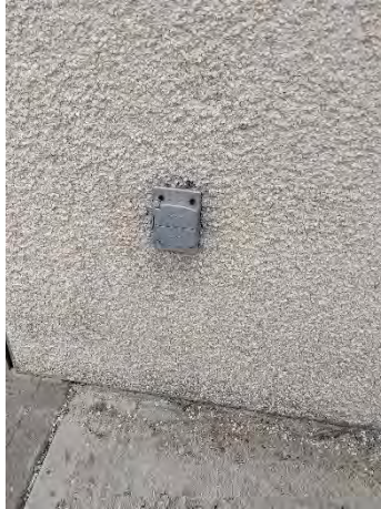
Figure 5-3 West Wing Main Distribution
