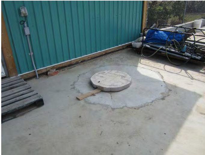
FIGURE 3 - New Sump Cover East of Richard Larson Remnant
