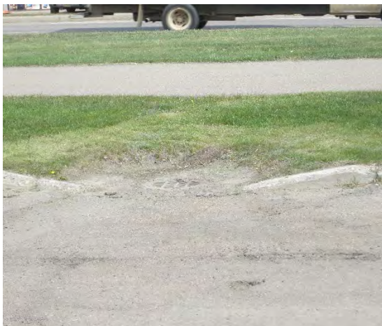
FIGURE 2 - Single Drain in Parking Lot for entire NE Site Area
