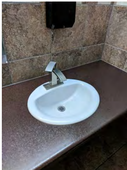
Figure 4-1 Typical LAV Found in Men and Women's Washroom by Main Entrance
