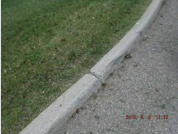
Figure 2-5 Parking Lot: Curbs with Edge Breaks
