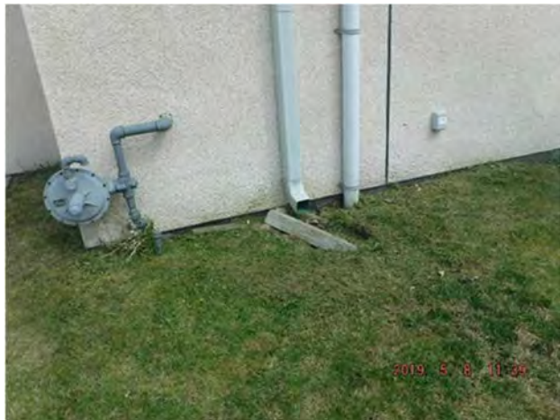
Figure 2-14 Misaligned Splashpads
