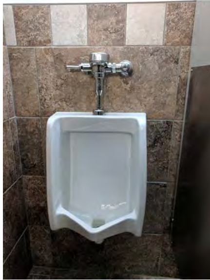
Figure 4-4 Urinal in Men's Washroom Near Main Entrance
