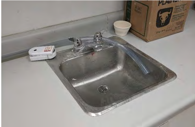
Figure 4-5 Sink Found in Kiln Room
