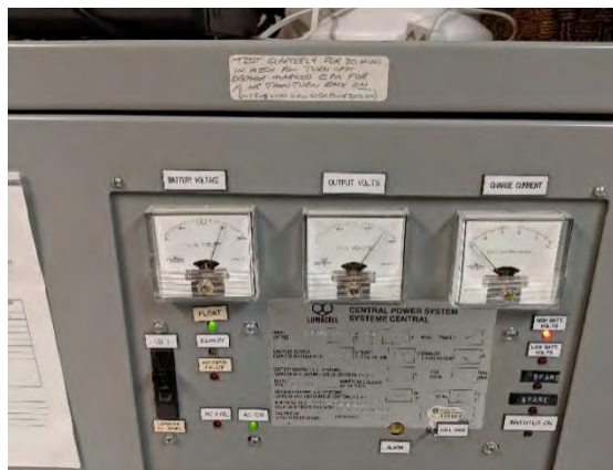
Figure 5-23 DC Inverter
