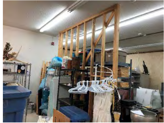
Figure 3-19 Temporary Timber Framed Supports
