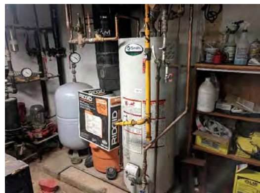
Figure 4-11 Gas Fired Domestic Water Heater System
