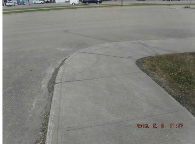
Figure 2-6 Parking Lot: Curbs with Edge Breaks
