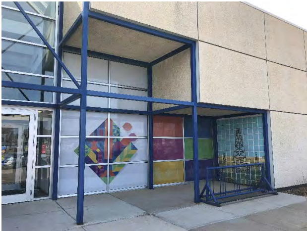
Figure 3-14 Viewing Main Entrance Framing
