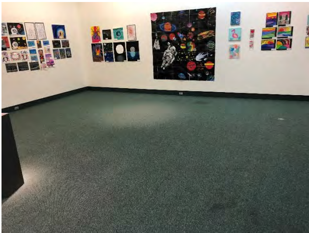
Figure 3-3 Floor Slab in Gallery Three
