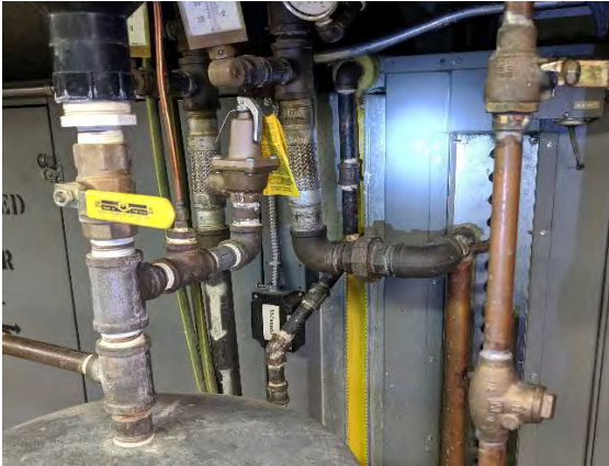
Figure 4-21 AHU-2 Heating Coil
