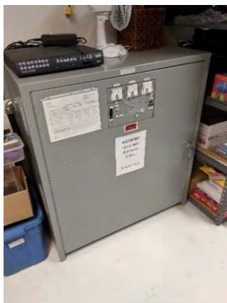
Figure 5-22 DC Inverter
