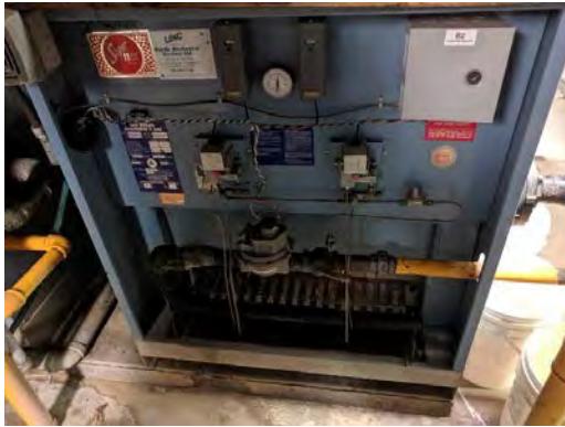
Figure 4-27 Typical B1/B2 Boiler
