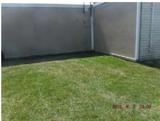
Figure 2-10 Back Graded: East Section (Fuchs gallery)
