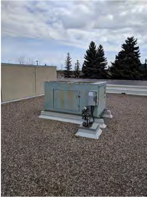
Figure 4-37 CH-1 on Roof
