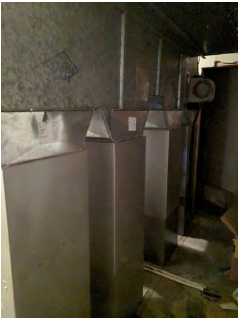
Figure 4-45 Fuchs and OTS Backside of Furnaces (Four Downdraft Furnaces with Humidifier in Back)
