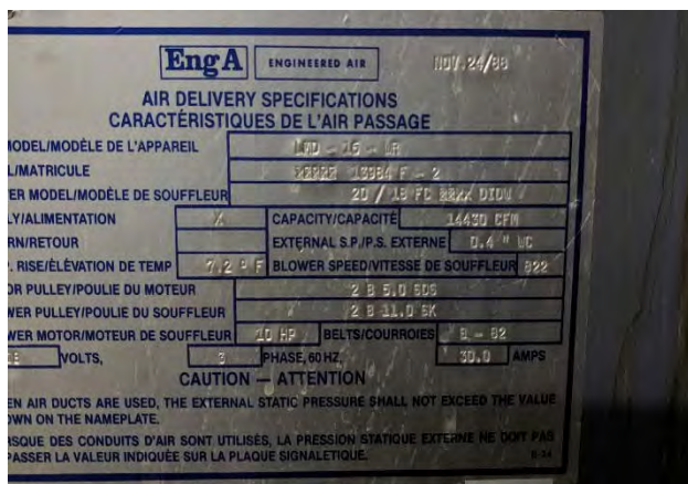
Figure 4-23 AHU-2 Nameplate
