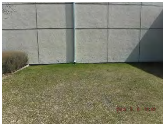
Figure 2-11 Insufficient Grading: West Section (Imhoff gallery)
