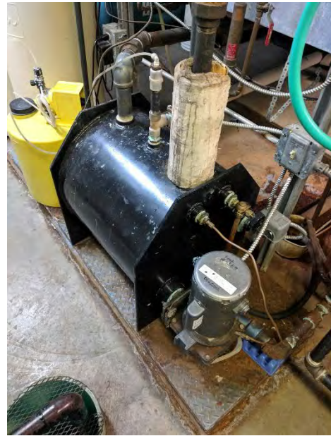
Figure 4-36 Condensate Collection Tank
