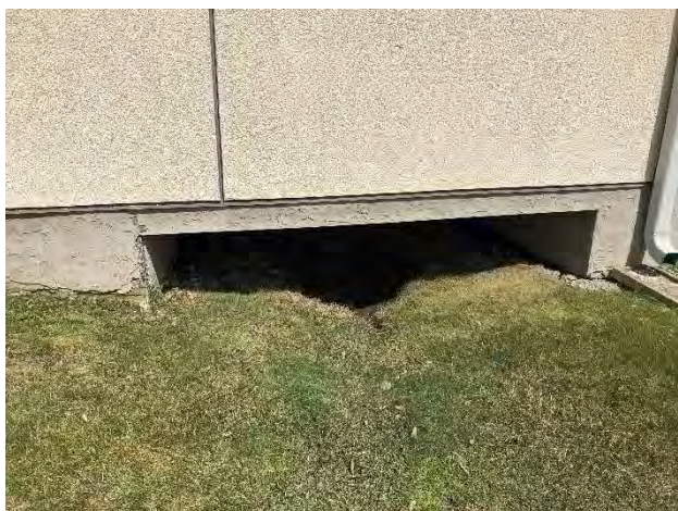
Figure 3-7 Corridor Link Suspended Slab
