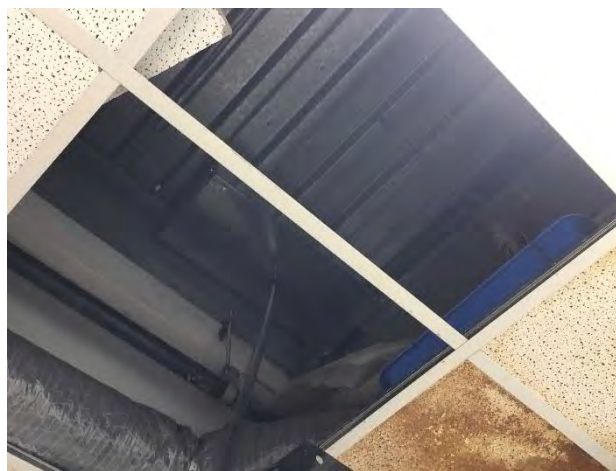
Figure 3-17 Viewing Condition of Roof Structure in Kitchen
