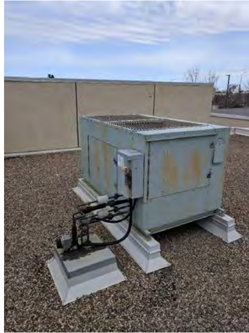
Figure 4-38 CH-1 on Roof
