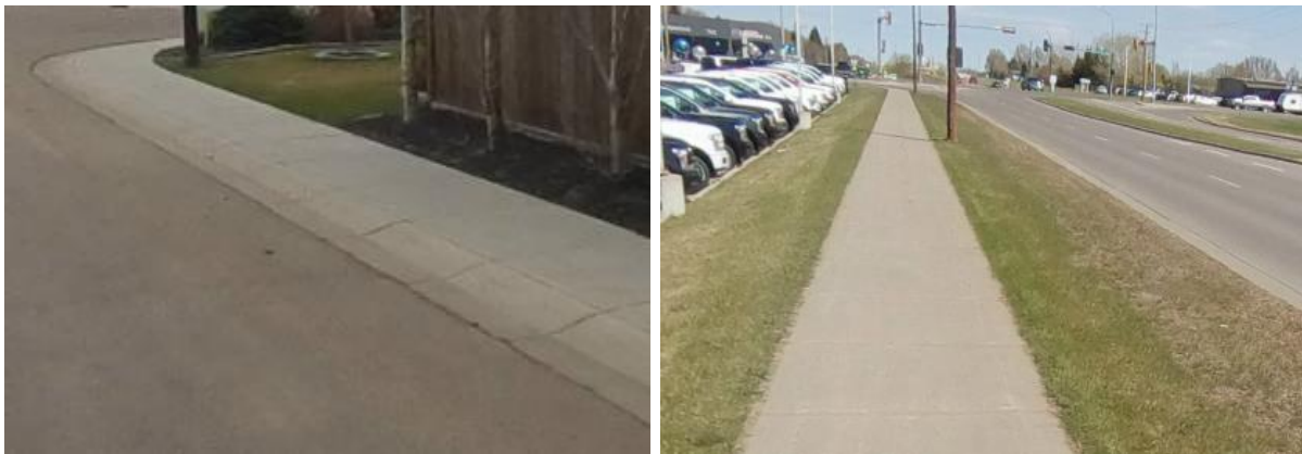
Examples of Sidewalks within the City of Lloydminster (mono-walk (Left), separated (Right))
