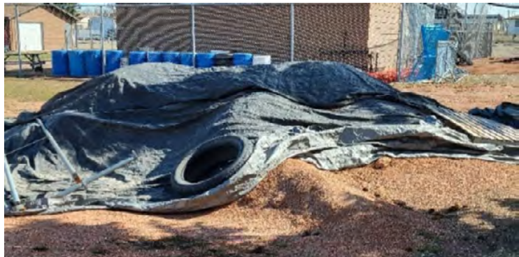
Shale and material storage for the ballpark was located adjacent to the maintenance yard but is only protected by tarps and tires. It is recommended that defined areas be created for material stockpiling and storage. Storing organic materials in this way could also contribute to organic waste reduction by composting and repurposing the materials on-site.
