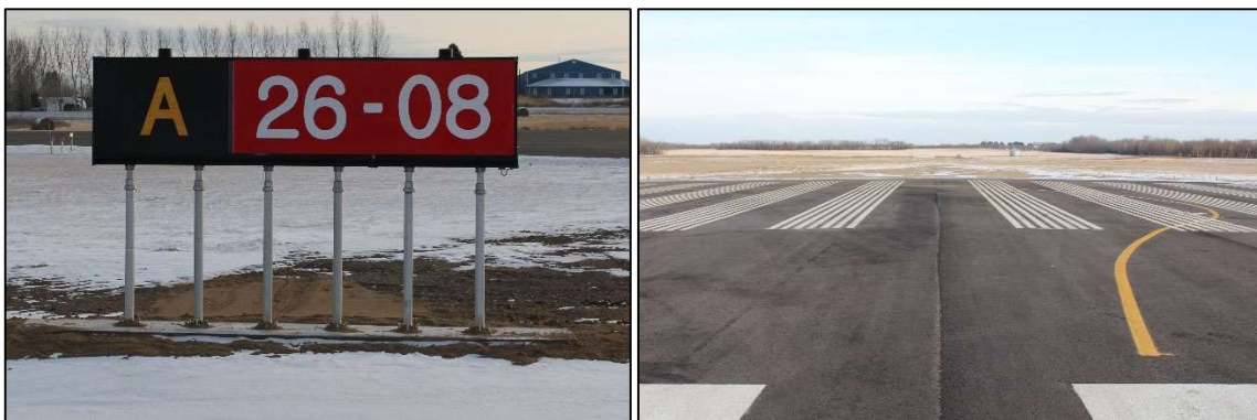
Runway 08-26 mandatory instruction sign (left) and pavement markings (right)
