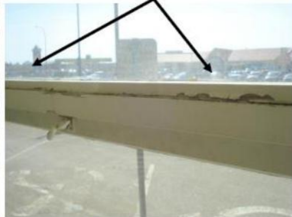
Photos 30 to 33: Moisture damages to interior sill and window frames
