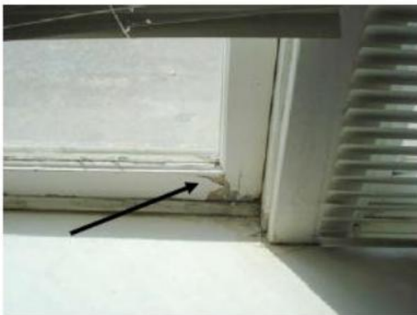
Photos 30 to 33: Moisture damages to interior sill and window frames
