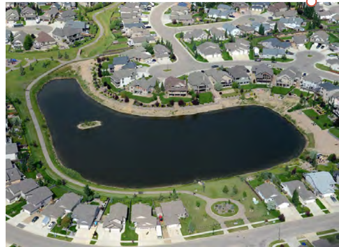
Stormwater management lake at College Park
