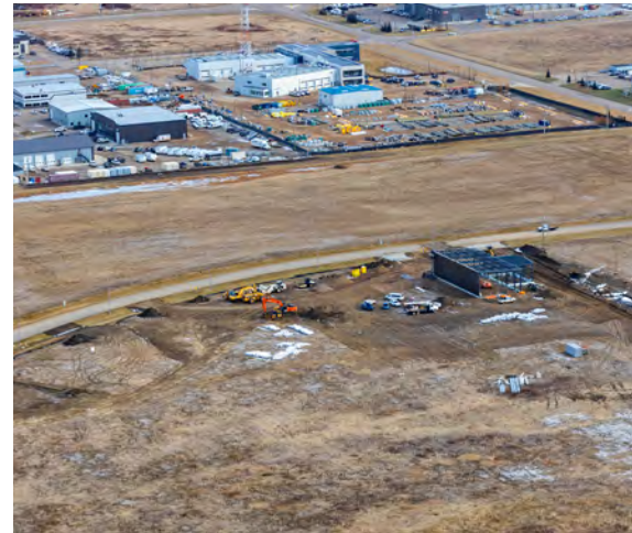
Aerial view of an industrial sector
