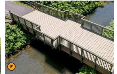
F NEW BRIDGE
