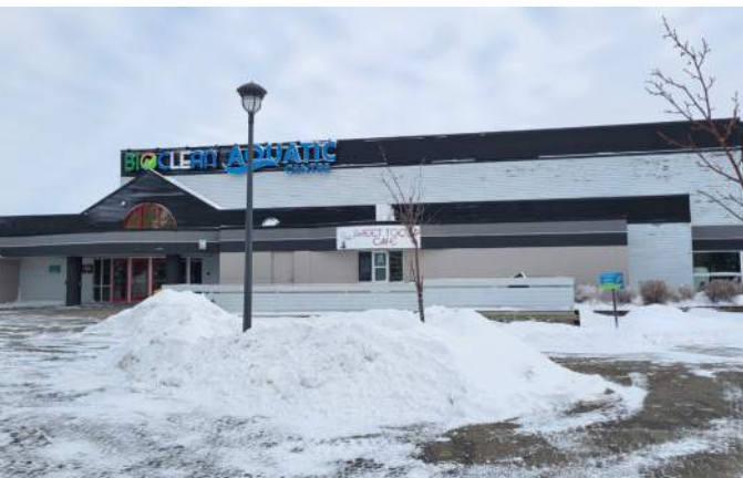
Existing BioClean Aquatic Centre
