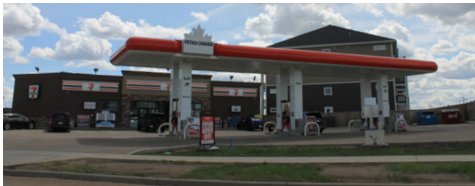
Figure 5-31. Neighbourhood Commercial Node A, 7401 34 Street
